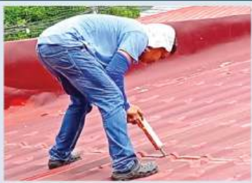
The roof of the school is repaired by applying roof sealant and fixing the gutter to prevent rain from leaking inside. This minimizes the risk of accidents caused by wet and slippery floors.
